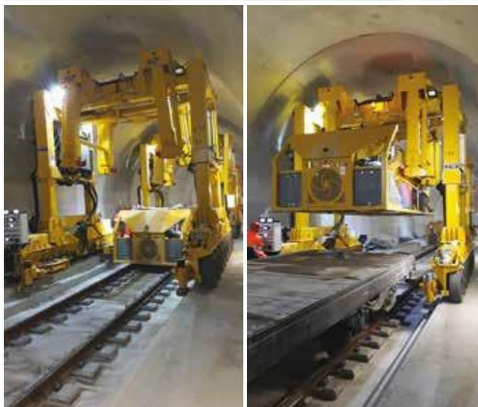
16A, 16B and 16C. The operating cycle for supplying concrete in the tunnel
