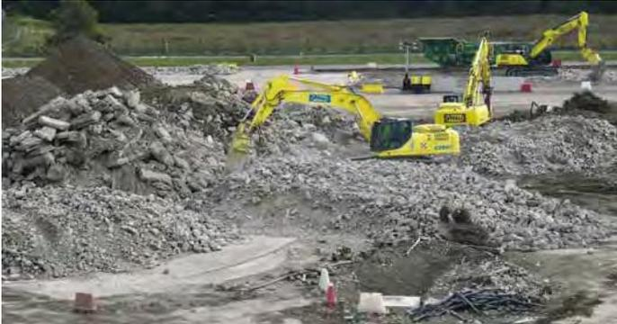
5. A specific zone was dedicated to processing demolished concrete for transformation in recycled aggregates.
