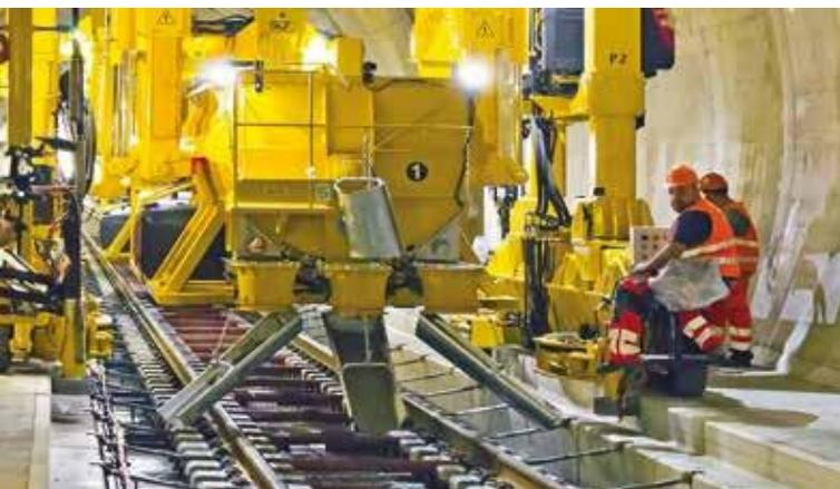
1. Concrete casting in the Monte Ceneri tunnel for GCF Spa for the Milan-Zurich high speed connection.
