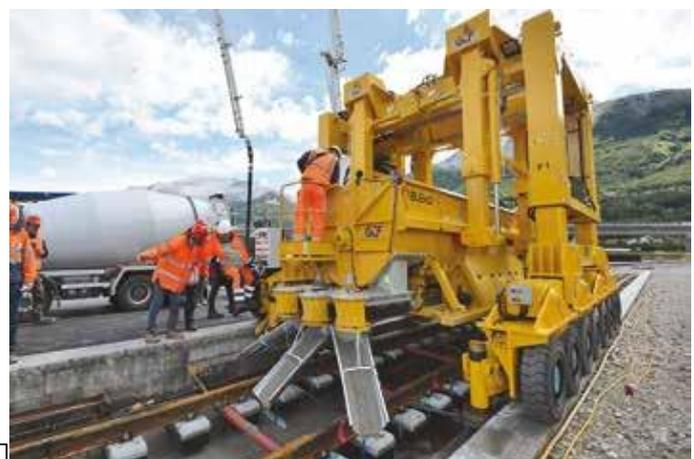
11. The unloading terminal specifically for the Monte Ceneri base tunnel proved highly efficient, allowing casts without having to protect the tracks.
